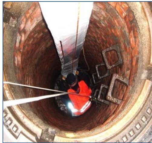
Liner winched in place ( NO scaffolding need )
